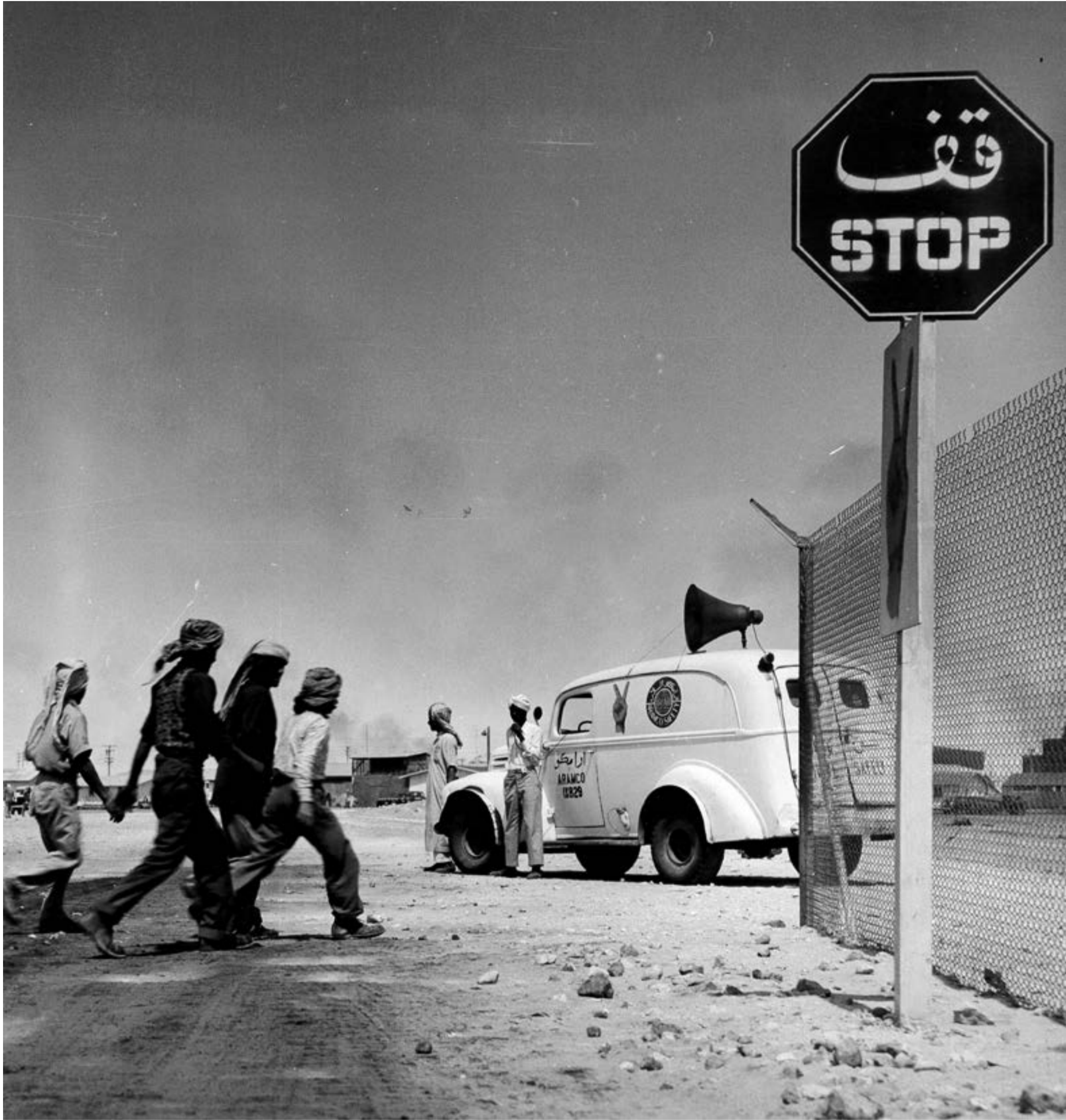
Before radio broadcasting was a possibility, other options were put to use. Here, a loudhailer mounted on a vehicle branded with the Aramco Safety logo makes safety announcements to passing workers.
